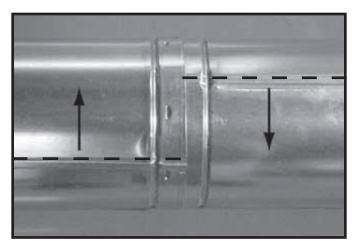
Figure 10.10 Rotate Seams for Disassembly
